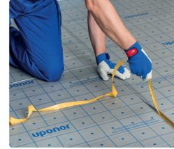
Self-adhesive strip along the panel for quick butt panels connection just remove the safety tape and connect the panels.
