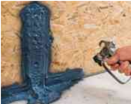
Airtight spraying over angle brackets,
